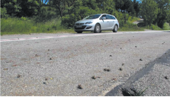
Figure 5: Route du col Bayard (24/06/2013). Photo: Marc Corail. Figure 5: Col Bayard road (24/06/2013). Picture: Marc Corail.
